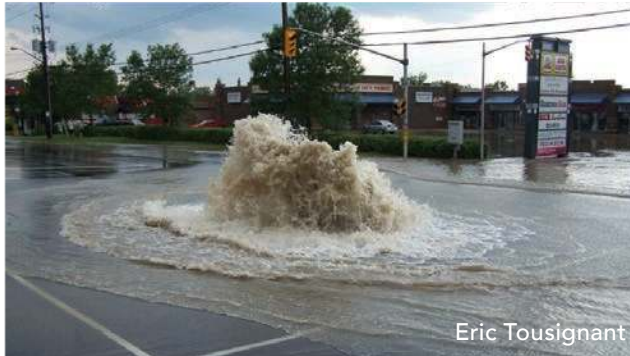
Storm sewer surcharging on St. Joseph Boulevard in Orleans, City of Ottawa (2006).
