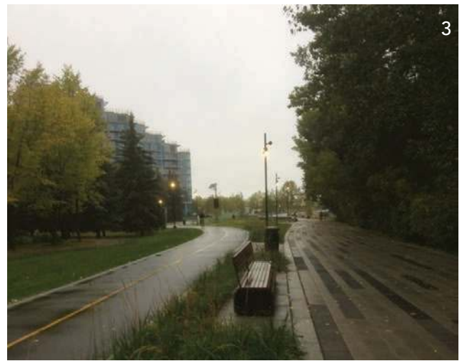
Figure 2 - Earthen berm portion of West Eau Claire Flood Barrier
